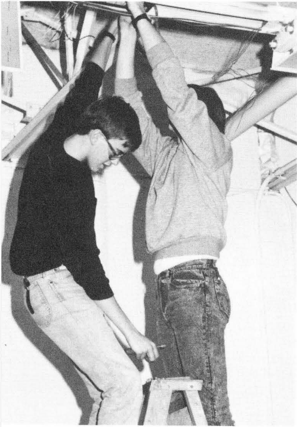
Working on electrical wiring, Mickey Potter reaches for a tool.
